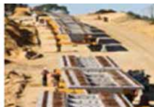
Bridge beams prior to installation
