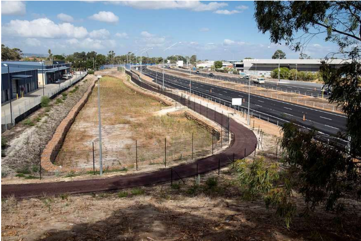
Image: vegetated infiltration basins
