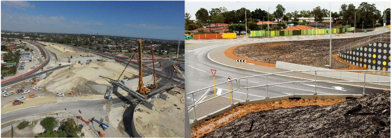
Image: Morley RAB beam lift and post completion
