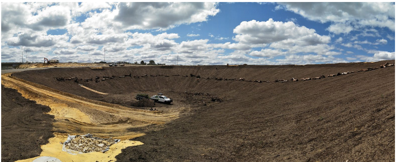
Figure 1 Fauna underpass in construction at MDC
