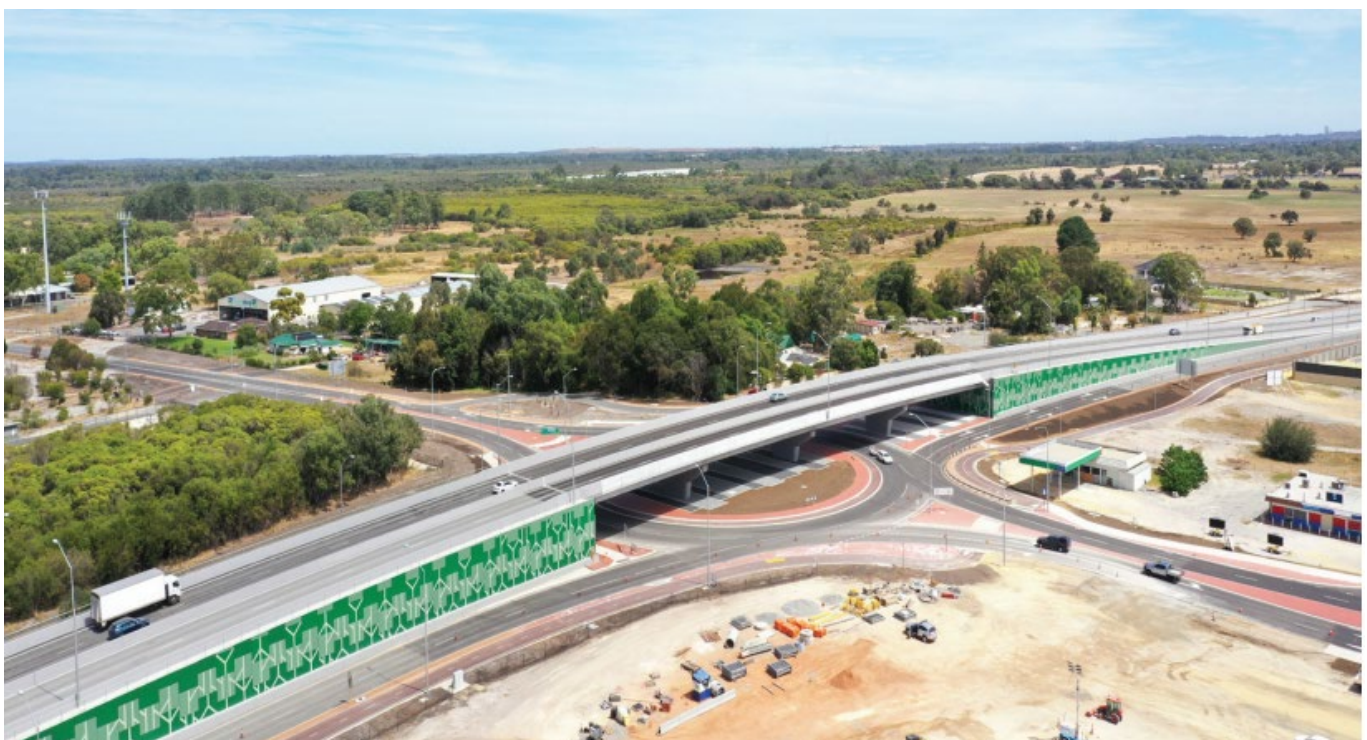
Figure 8 Bridge over Nicholson Road, March 2020
