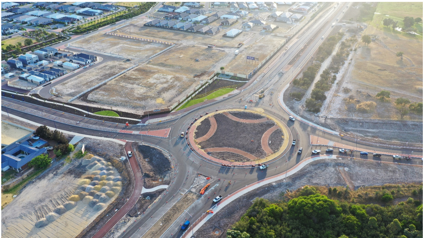
Figure 5 Taylor Road – Wright Road intersection at ARU
