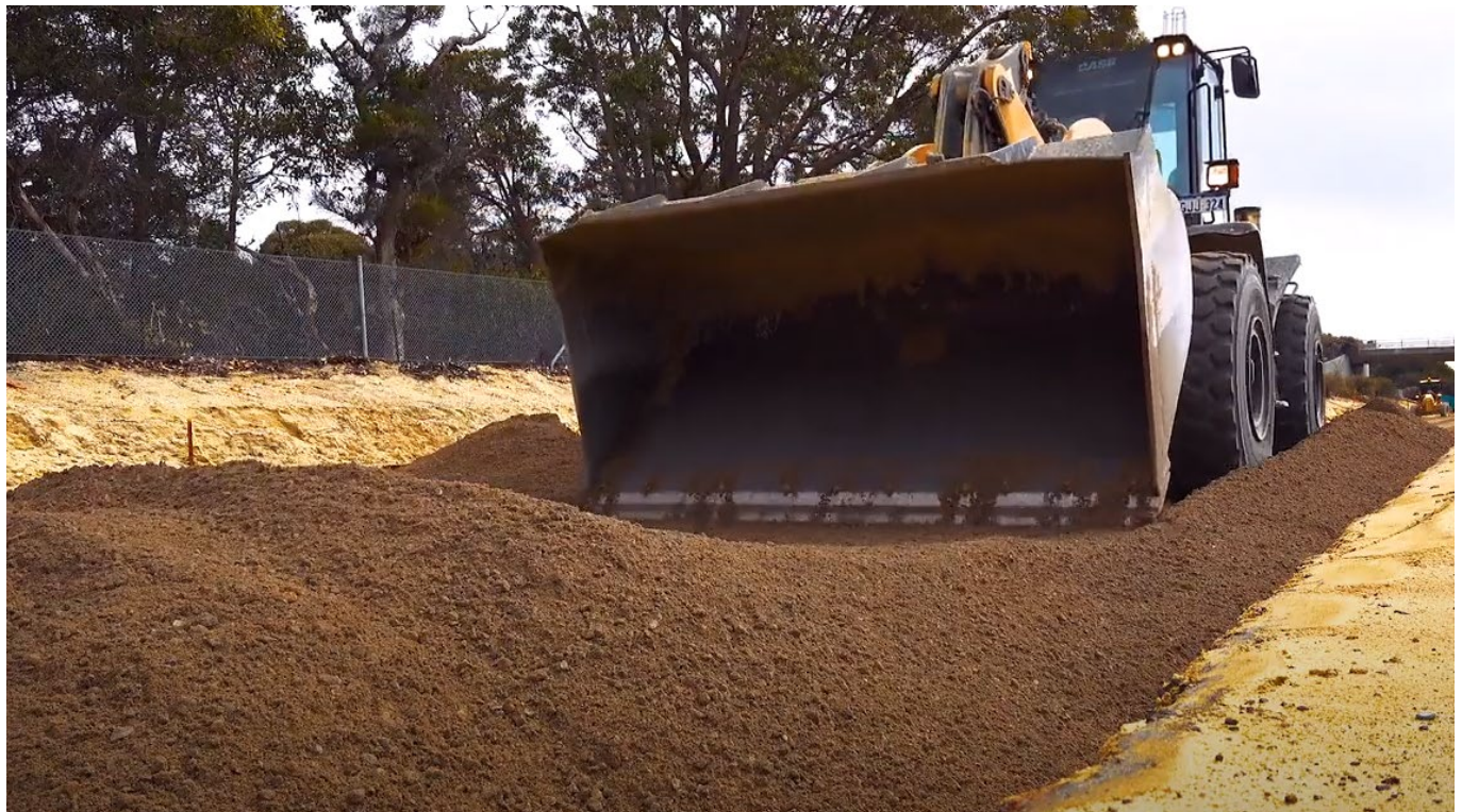
Figure 3 Crushed recycled concrete used on Murdoch Drive Connection
