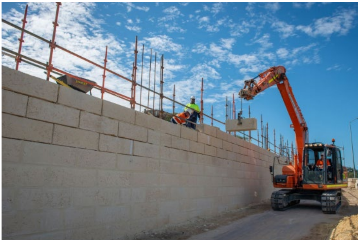
Figure 7 Leeming noise wall construction, October 2019
