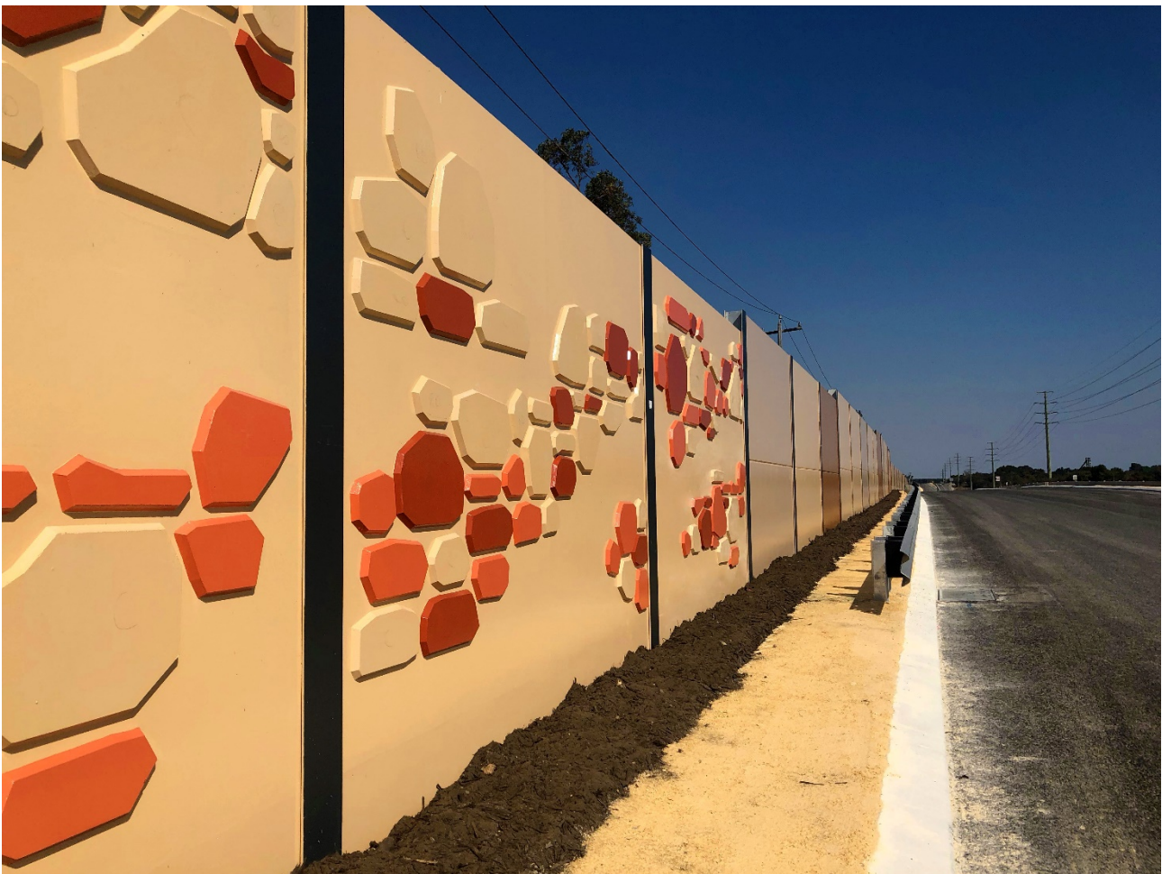
Figure 4 Noise walls along Wanneroo Road
