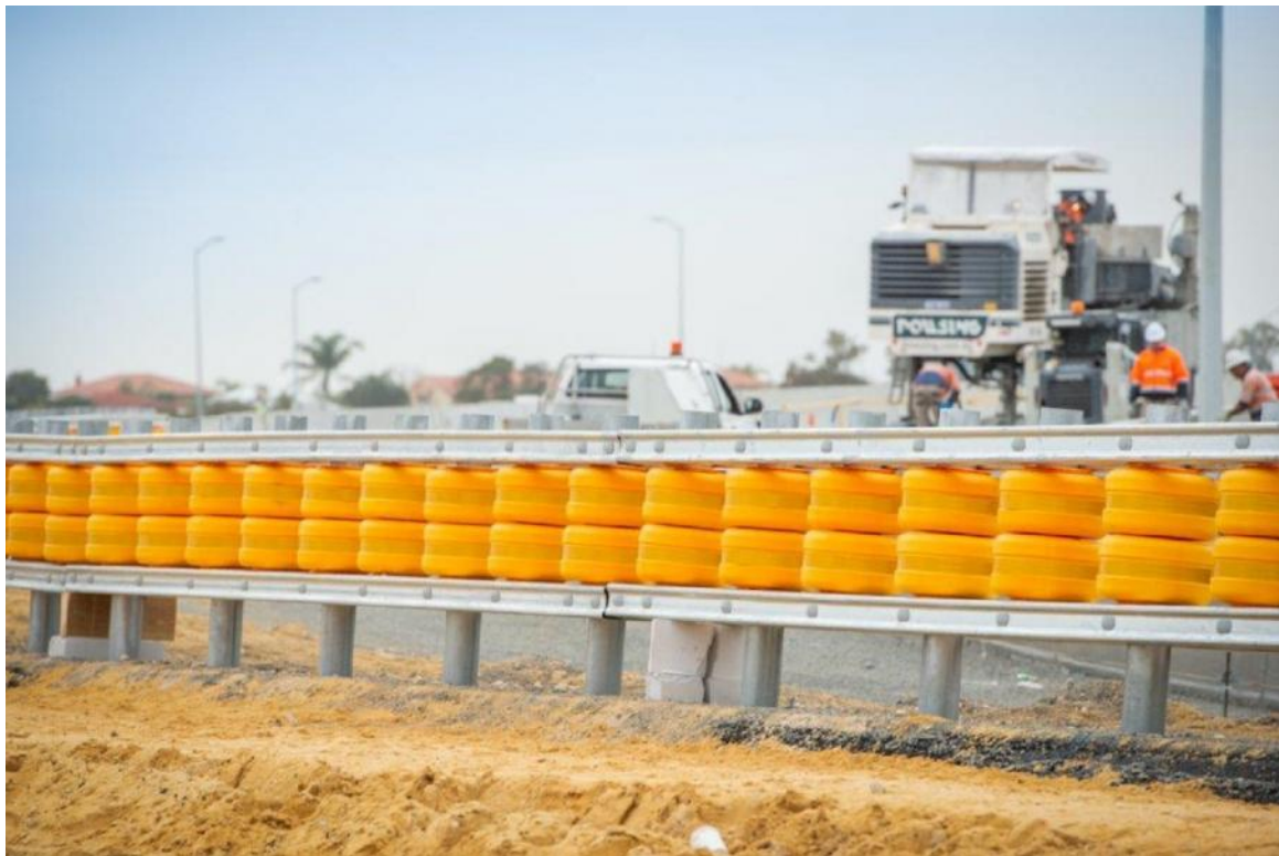
Figure 10 Roller safety barriers on Murdoch Drive Connection ramp, August 2019
