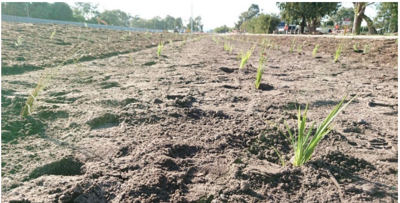
Figure 11 Landscaping underway at ARU, February 2020
