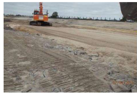
Figure 3: 300mm lift track rolled 4 passes.
