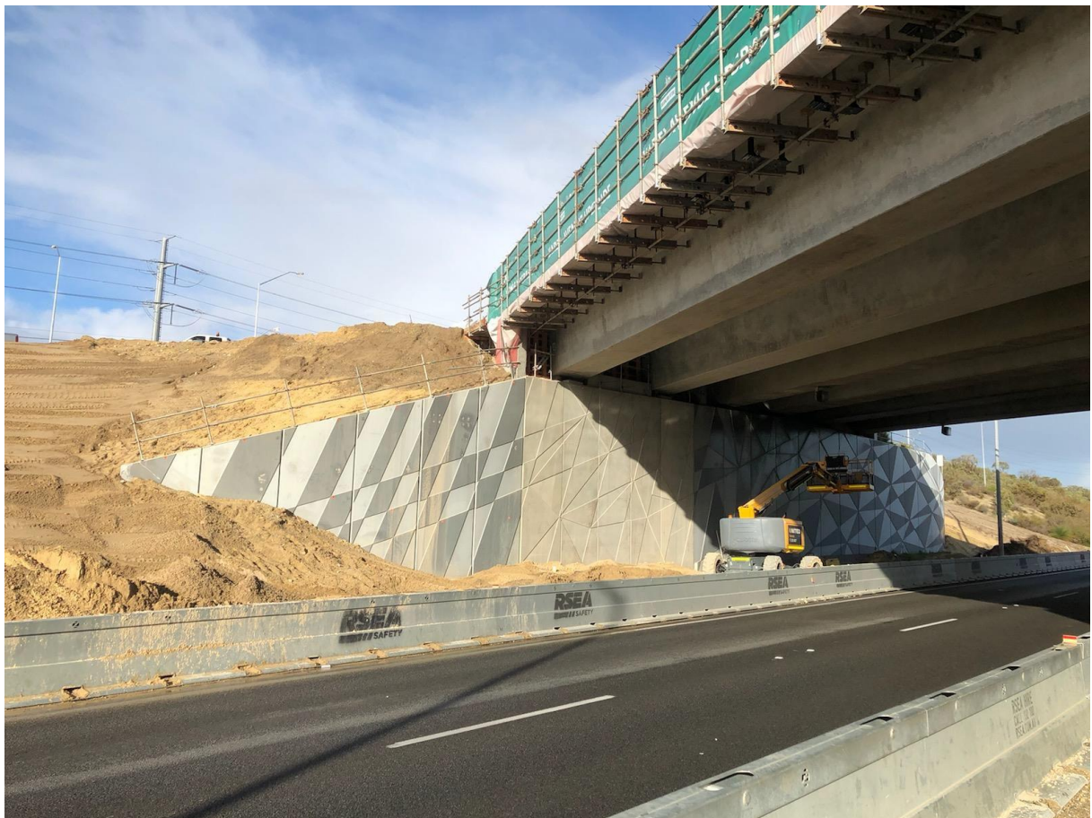
Figure 5: Re-used Wall Panels for Bridge 1857 (See the panels to the left of the unpainted five panels)
