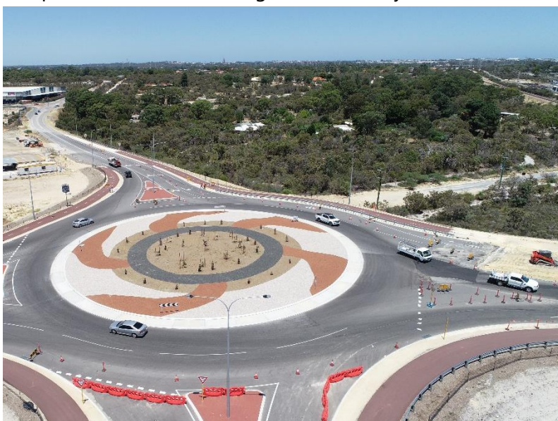
Image 4: Aerial view of Berriqan Drive roundabout during construction
