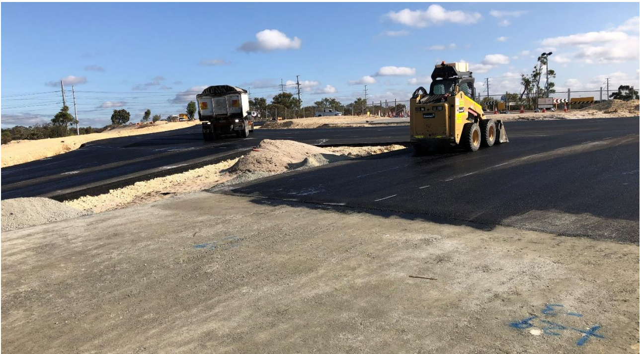
Image 1: CRC under FDA during construction
