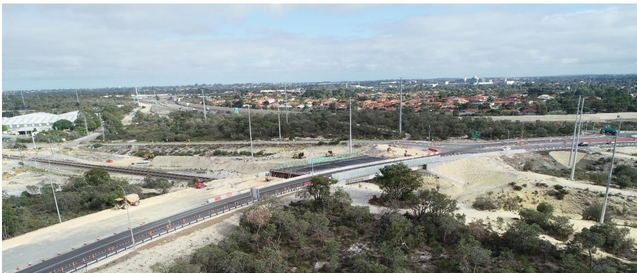
Image 5: Visual of Bridge over rail, and residential area in the background.
