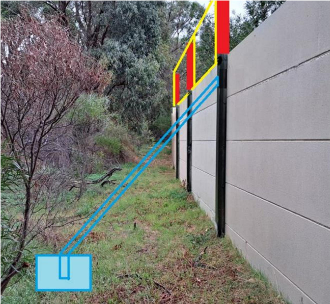
Figure 4 Contingency Back Stay, Should Existing Footing not Meet Future Wind Loading Requirements
