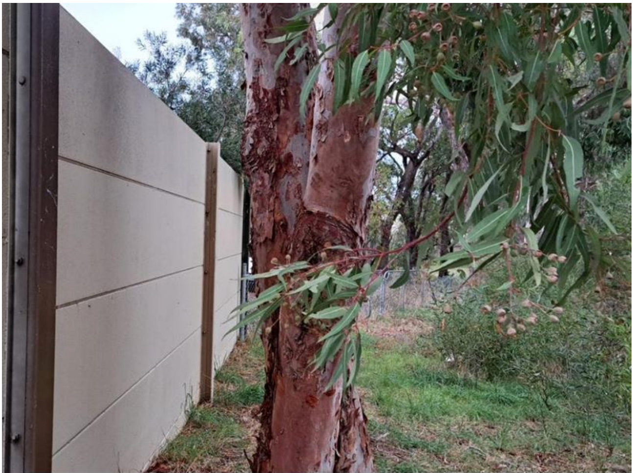
Figure 2 Existing Noise Wall Structure (NW17)
