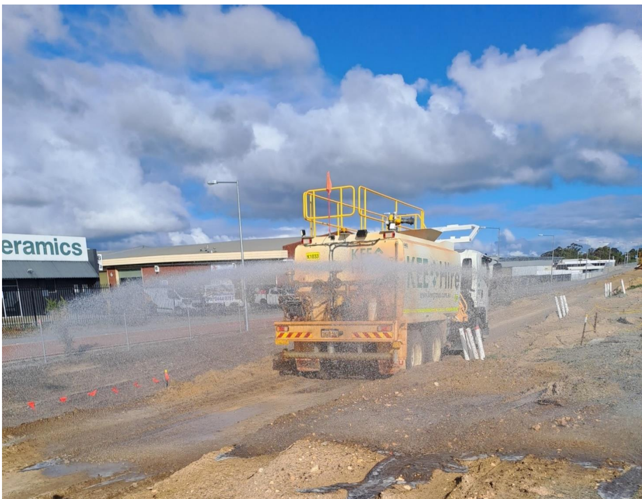
Figure 8 Water Cart On-Site in Operation
