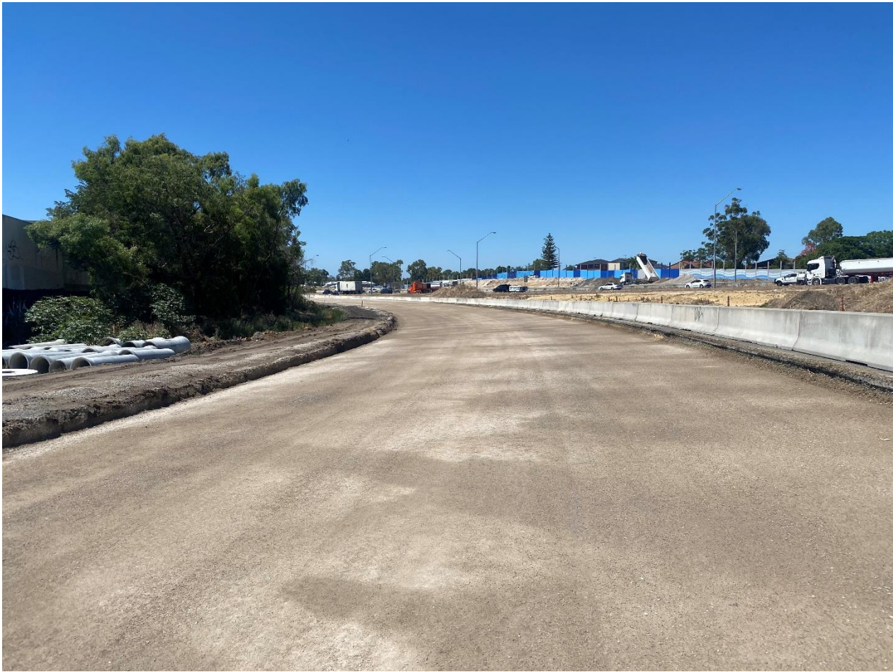
Figure 13 Crushed Recycled Concrete subbase placed onsite
