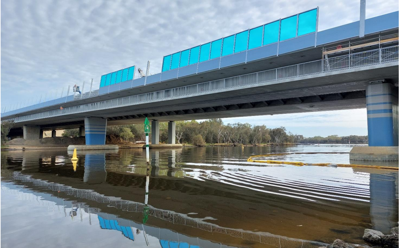
Figure 17 Installation of noise walls on Redcliffe Bridge
