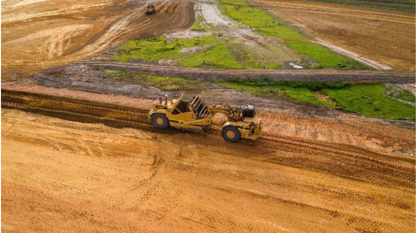
Image 3 Scraper at ramp 3 – materials won stockpiled for use on Project
