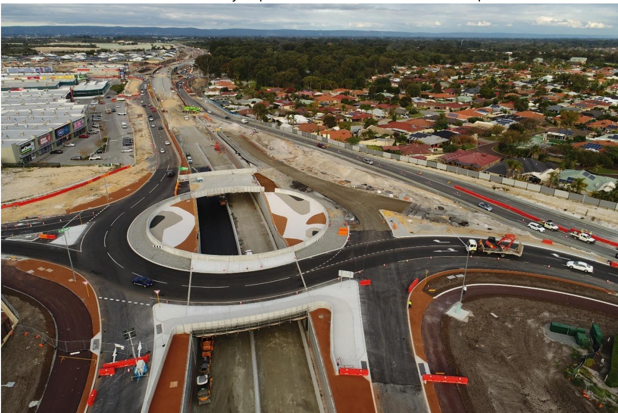
Figure 13: Solomon Road Roundabout/Dive Structure Progress
