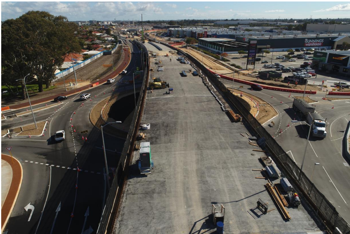
Figure 6: Tapper Road – Verde Drive Bridge Progress
