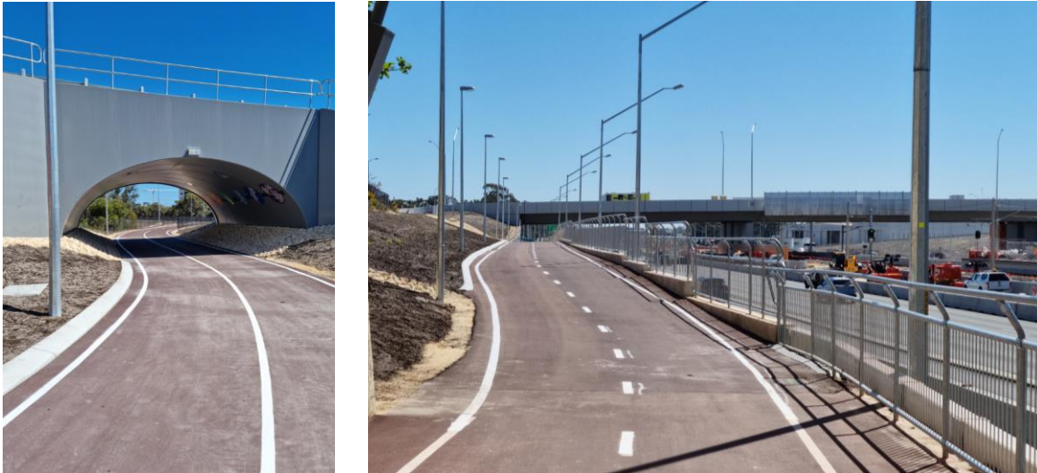
Figure 12: PSP – west of Kwinana Freeway Progress
