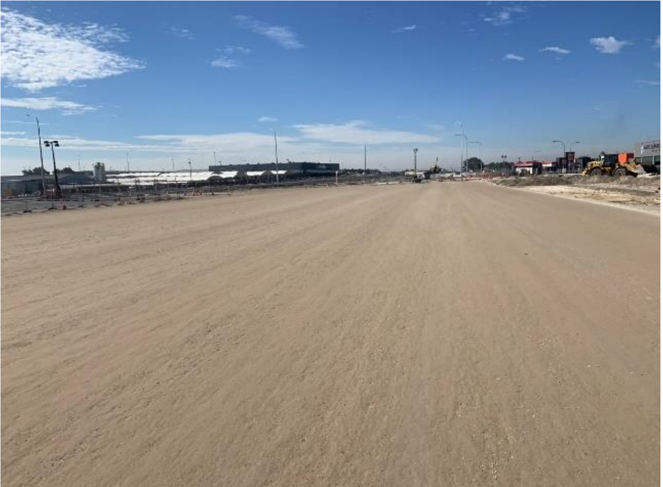
Figure 9: Crushed Recycled Concrete Subbase complete after trimming and sweeping
