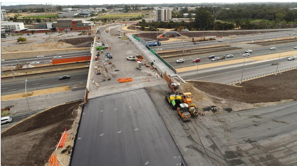
Figure 2: Armadale Road to North Lake Road Bridge Progress
