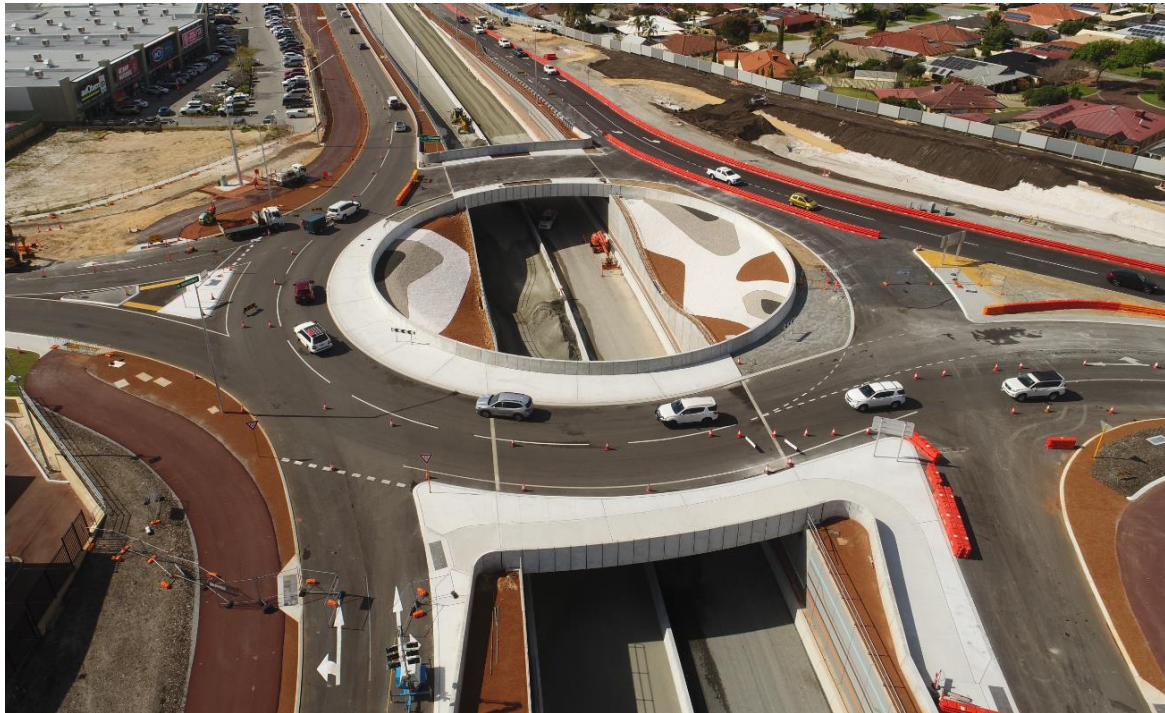
Figure 5: Solomon Road Dive Structure Progress
