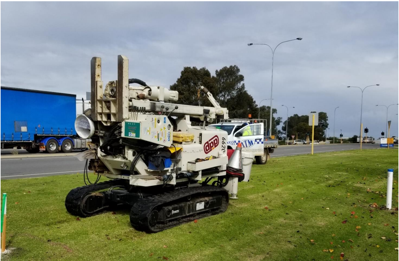
Figure 4 drill rig to be used during dewatering and excavation construction processes.
