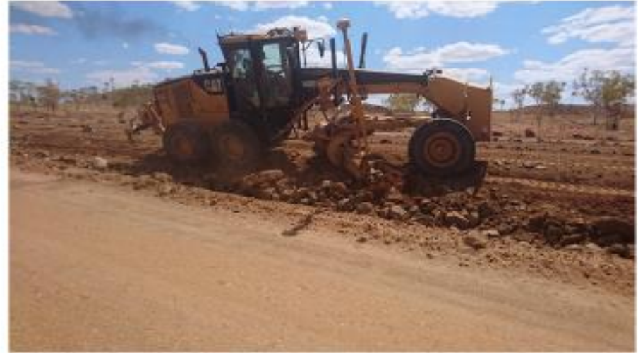
Heavy vehicle turnaround installed
