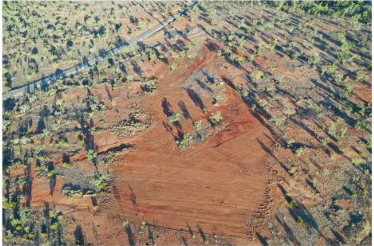
Batch Plant Location after Decommissioning of Section 1.0
