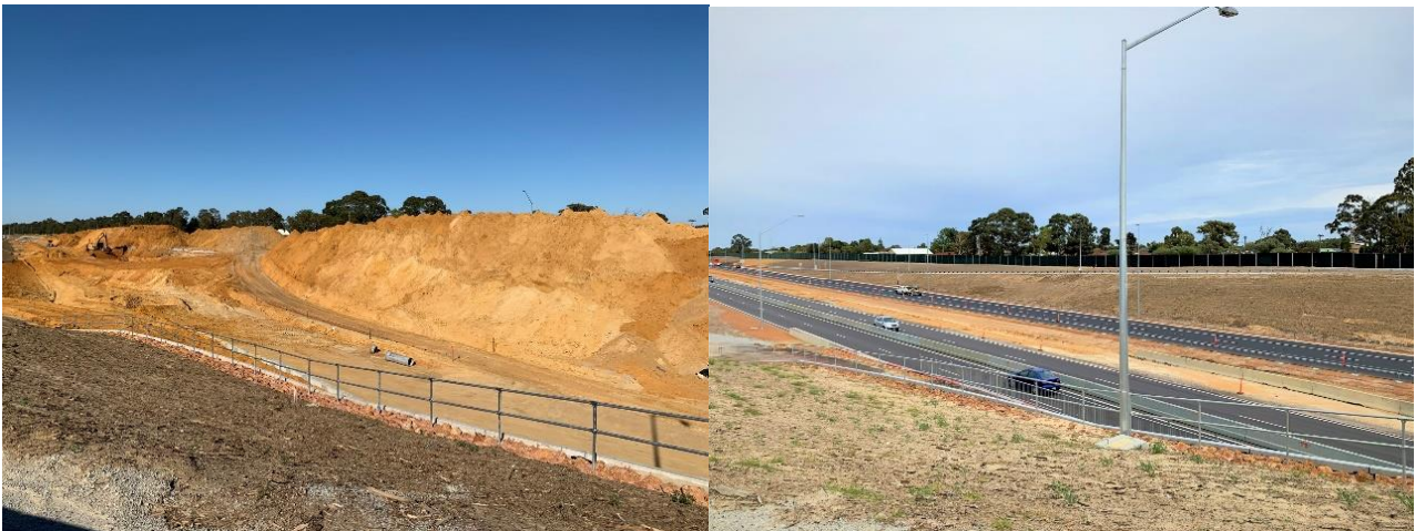
Images 2 & 3: Roe Highway before and after excavations
