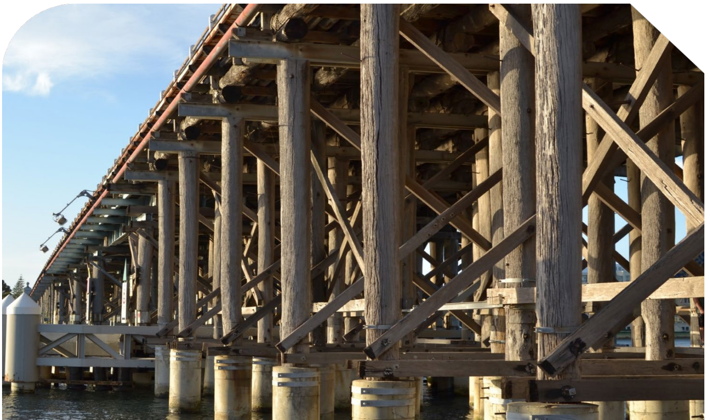
Figure 3 Fremantle Traffic Bridge piers
