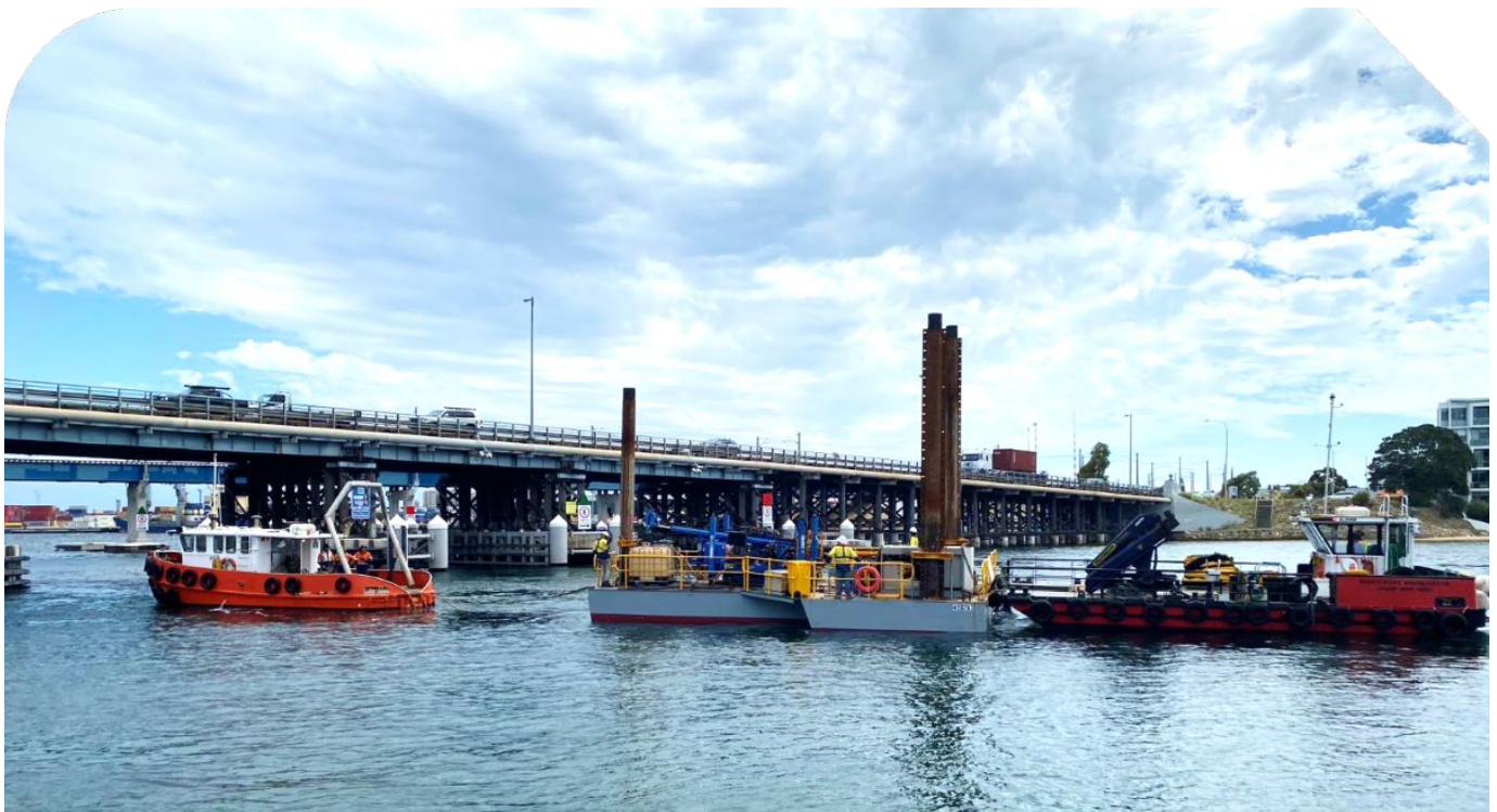
Figure 12 Swan River Crossings in-river geotechnical investigations
