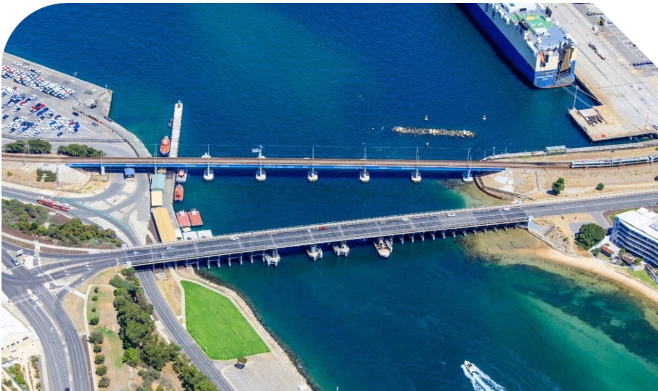
Figure 10 Aerial image of the existing Fremantle Traffic Bridge and rail bridge (looking west to Indian Ocean)
